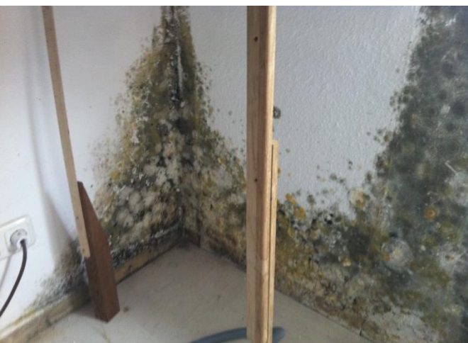
Massive mould damage behind a removed kitchen range
